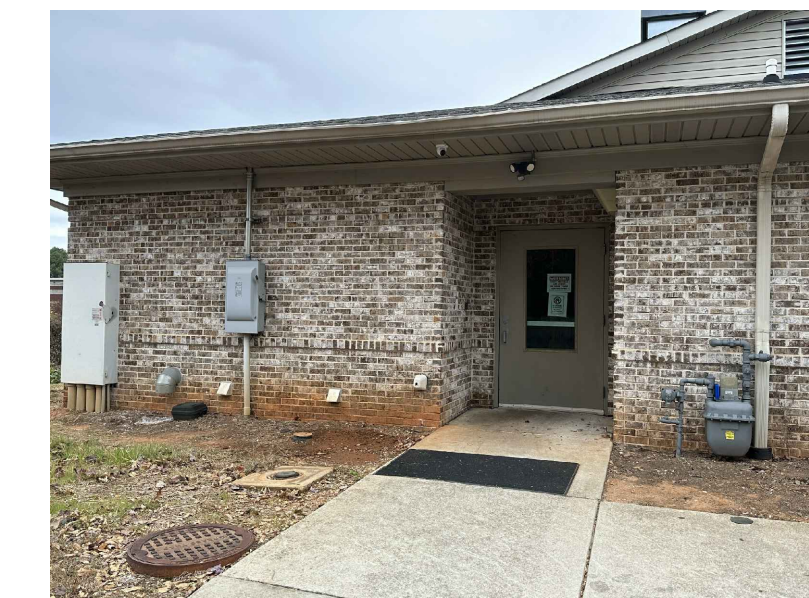
7. SERVICE | Kitchen Entrance
