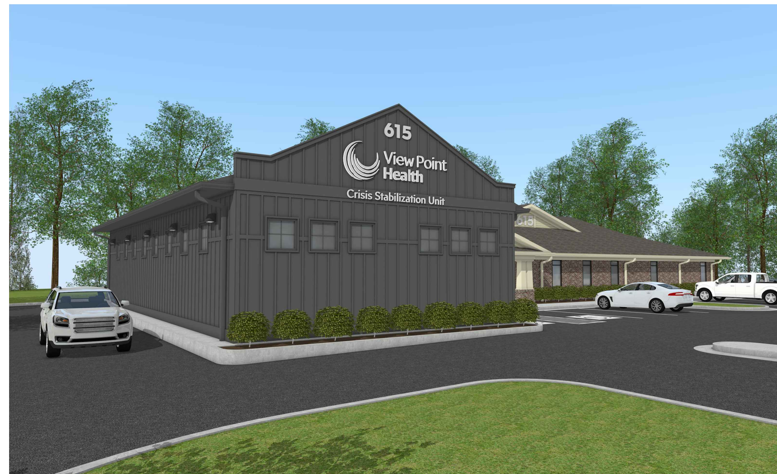
3 | Front Facade View
